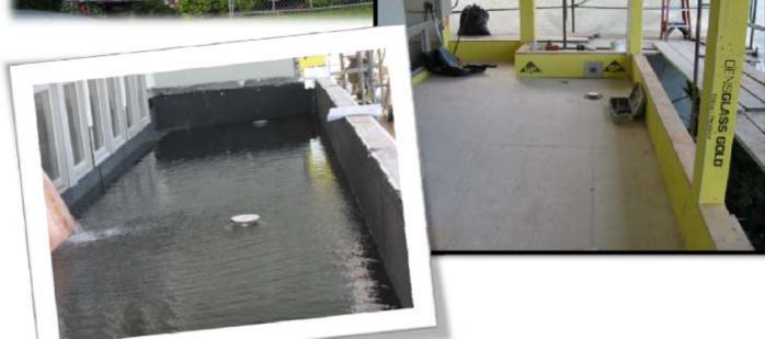
Cobra Construction worked with a local engineering firm and this HOA to correct faulty workmanship performed by the previous repair contractor. Work included: Structural framing repairs; installation of a new deck waterproofing system, which required the decks to hold water over a 24-hour period to demonstrate its water tight seal; installation of bi-folding Nana Doors; selective stucco repairs; new sheet metal coping; and the installation of new glass panel railings.
